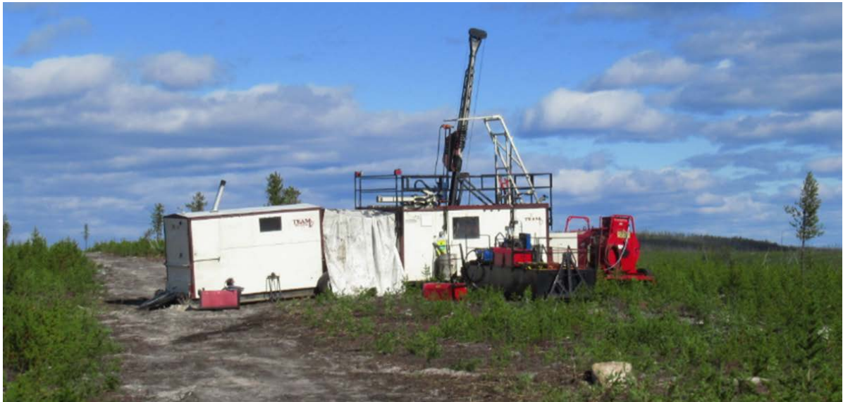
Figure 17: Team Drilling Limited Drill Rig During the 2018 Summer Drilling Program
